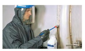
Avesta Pickling Gel 122 is easy to apply thanks to its free-flowing consistency.
